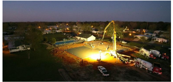
Pouring cement at sunrise
